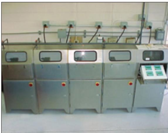
Mixed oxidants, produced by generators such as this one, have the disinfection power of chlorine and have also been documented to inactivate even chlorine-resistant microorganisms.
