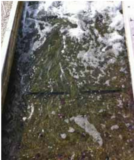
The onsite generation system eliminated visible algae from the distribution deck.
