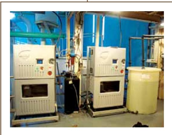
The Cedar Knox plant's electrolytic cells self-clean after 700 hours of operation, reducing maintenance needs.
