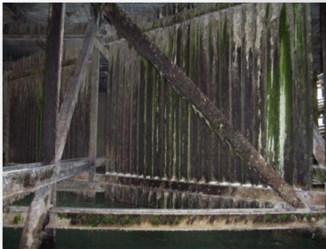
Biofilm with conventional biocide program
