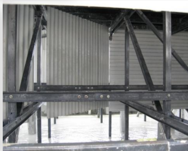
Biofilm eliminated with mixed oxidants
