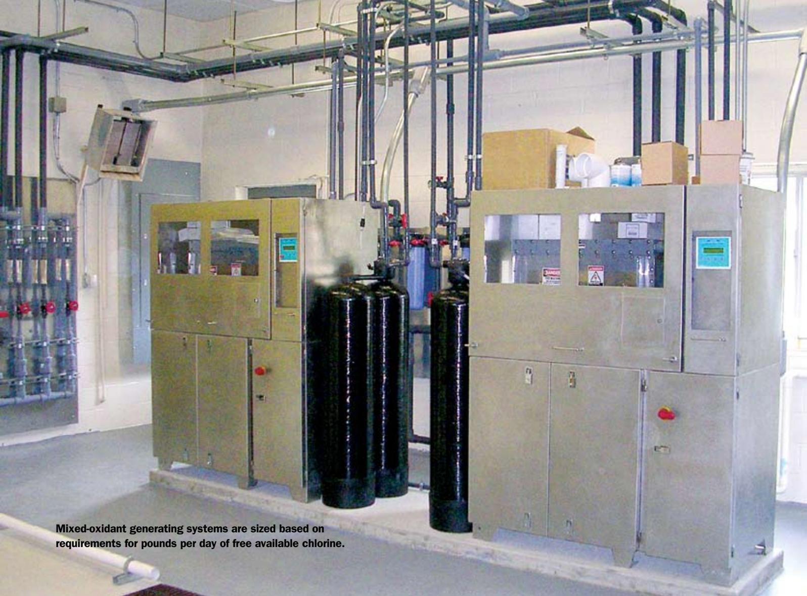
**Mixed-oxidant generating systems are sized based on requirements for pounds per day of free available chlorine.**
