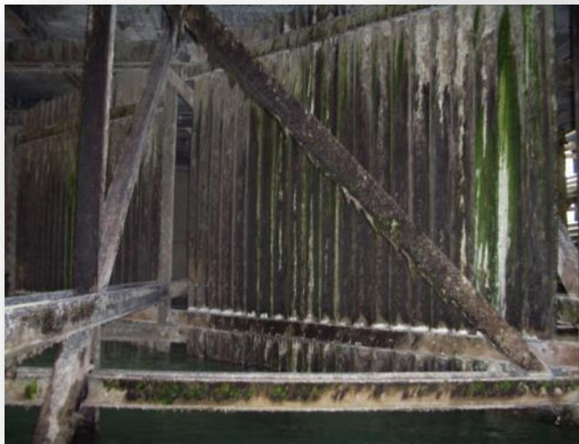
Biofilm with conventional biocide program
