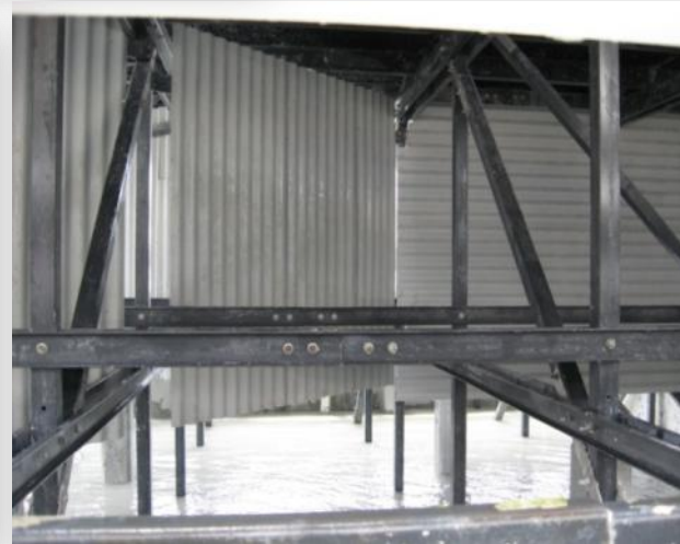
Biofilm eliminated with mixed oxidant solution
