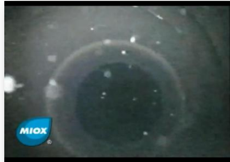
Filter recirculation pipe 22 days after mixed oxidants
