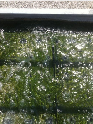
Distribution deck before MIOX® : visible live green algae
